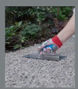
Use a ratio of 1L of Gravel Grip to 25kg of aggregates.
